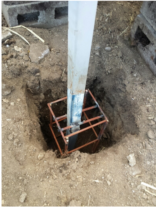
Typical footing excavation for Operators Hut
